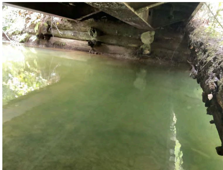
Right Bank Abutment when facing downstream
