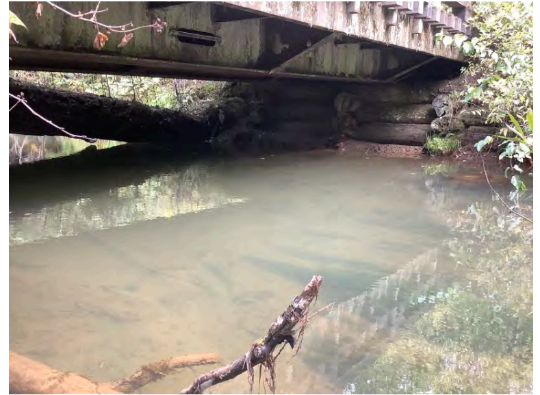
Left Bank Abutment when facing downstream
