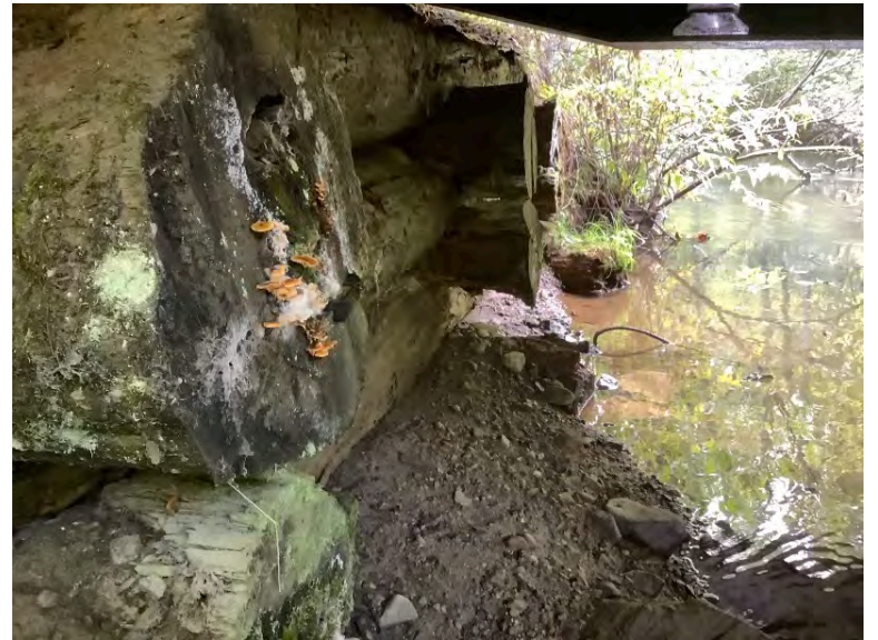
Left Bank Abutment when facing downstream
